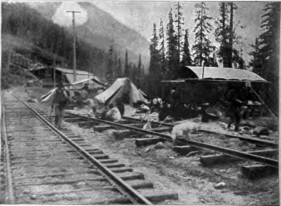
RAILWAY CONSTRUCTION IN THE MOUNTAINS.
